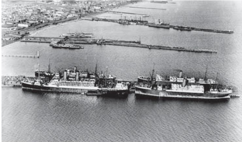
Aerial View of Port Melbourne Piers circa 1926 when Station Pier (centre) was under construction. Public Record Office Victoria, VPRS 12800 P1, H1239.
